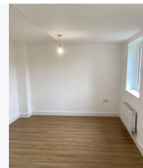
Ref # 7.5 - White painted plaster in lounge
