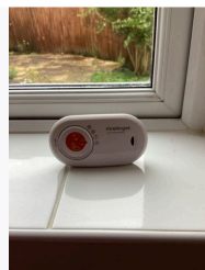
Ref # 4.3 - Carbon monoxide alarm - on kitchen window sill
